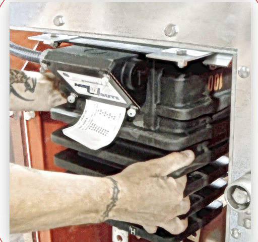
Slide-in CT stainless steel mounting hardware allows for ease of installation or removal
